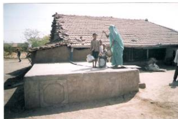
Construction of Roof Rainwater Harvesting Tank
